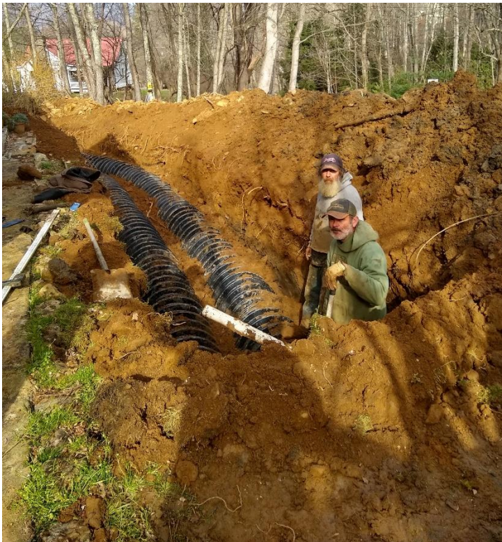
Installing septic field drain lines
