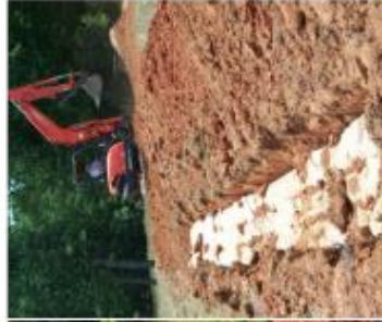
The drain field must be installed level and on contour with the landscape.
