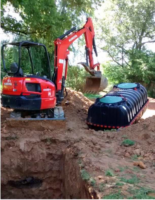
Installing septic tank
