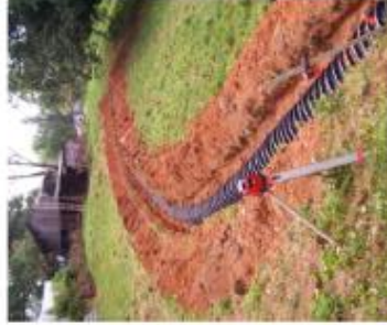
The drain field must be installed level and on contour with the landscape.
